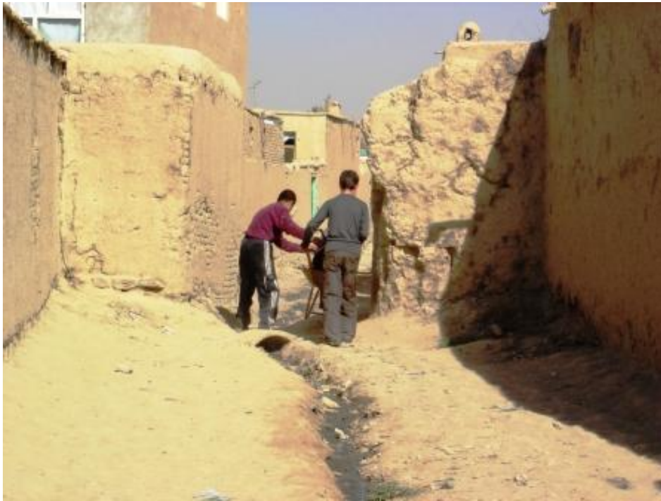
Figure 3: A Passage-Way Before Upgrading
