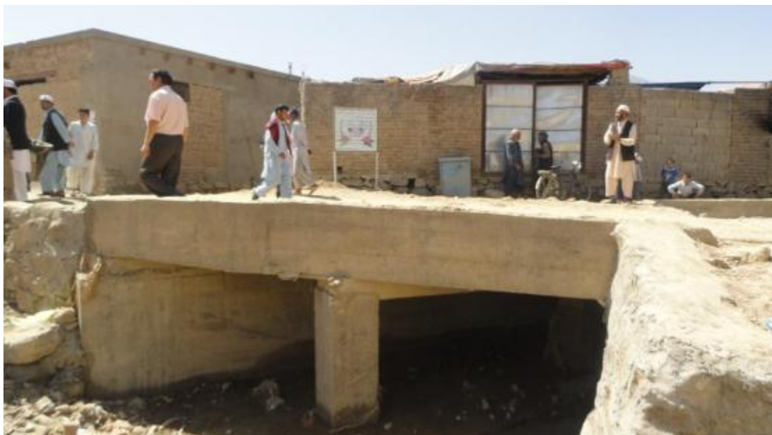
Figure 5: Culvert Constructed through Conditional Small Grant to Dough Abad in District 13
