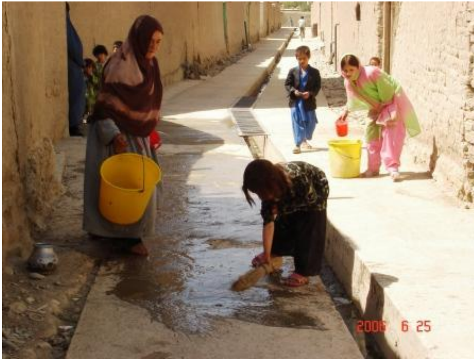
Figure 2: Community Council Members and Families Curing the Concrete
